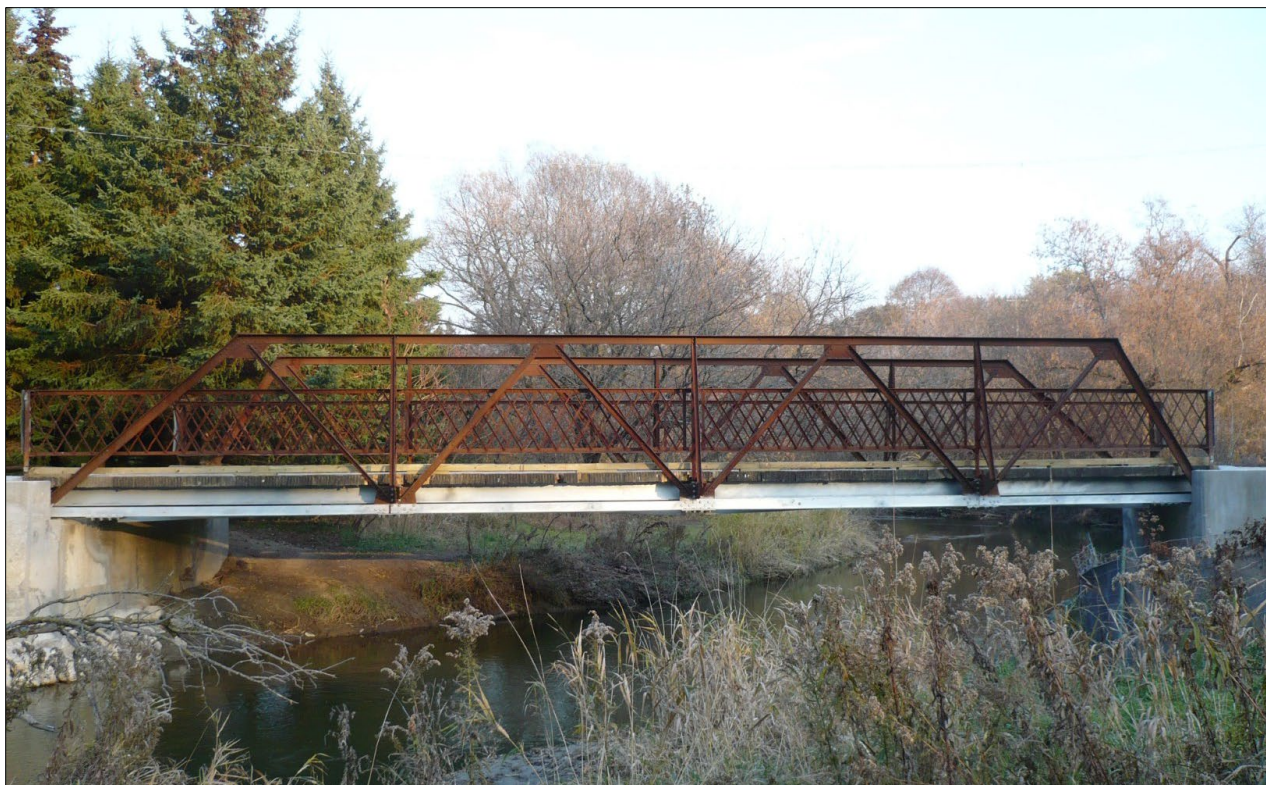
Sneath Road Bridge – Town of Caledon. Deck and every truss element below the deck was replaced. Foundations were repaired.
